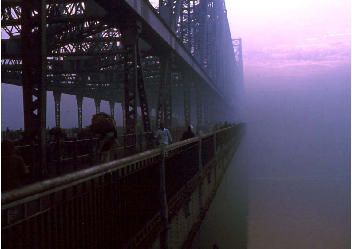
Howrah bridge, Calcutta
